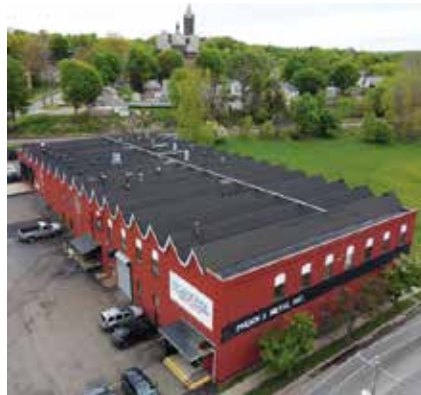
Historic saw-tooth configuration prior to slope build-up installation.
