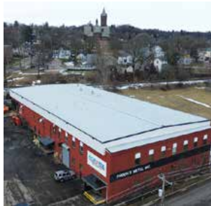
Finished double-slope configuration replacing original saw tooth geometry.
