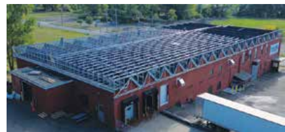
New structural framing installed above existing saw-tooth roof without demolition.
