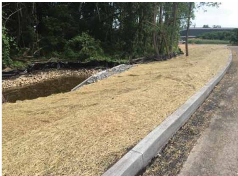
Proper Construction Phase: Rolled straw seed blanket installed following final grading of topsoil.
